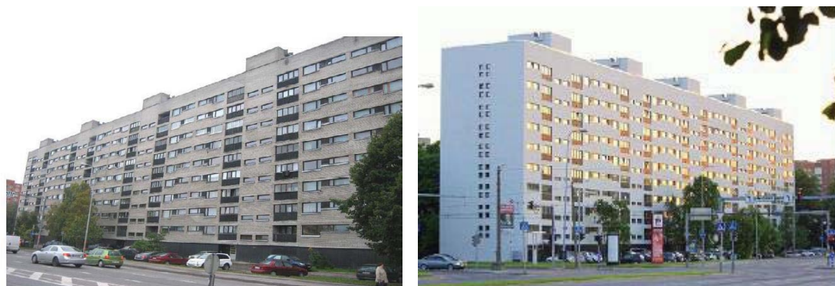
Figure 58: A financed project example- renovation of the apartment block in Tallinn (before and after)
