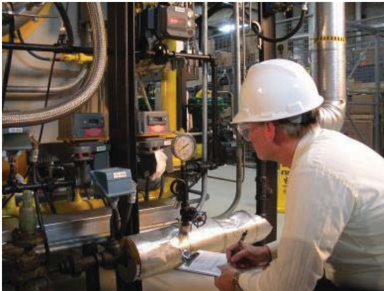
Figure 33: Energy auditor at work
